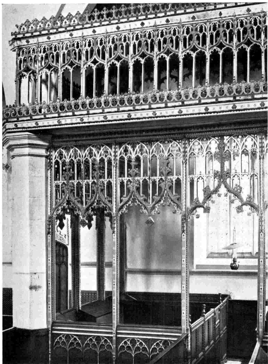
DENNINGTON. North Parclose. 15th Century. A "restoration."
